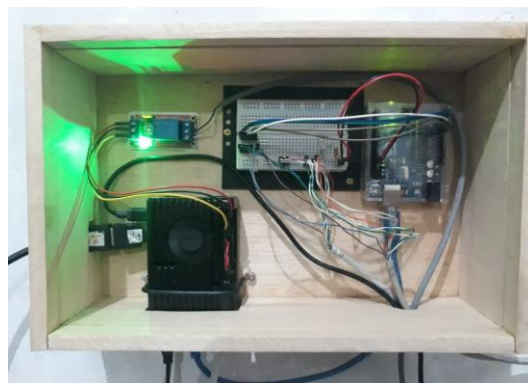
Fig. 2. The equipment assembly
